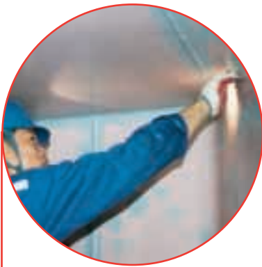
Inspection of stripe coats.
