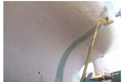
Intersleek® tiecoat being applied
