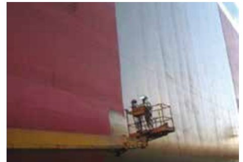
Application of Intersleek® Linkcoat
