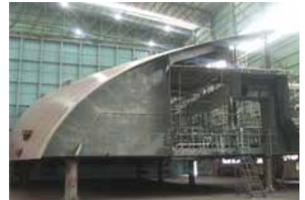
Intergard 7500 applied to a water ballast tank
