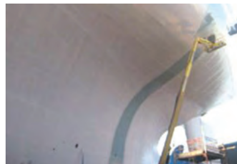
施工Intersleek®过渡涂层
