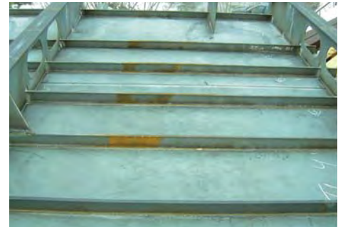
Interplate®Zero has excellent anticorrosion properties
