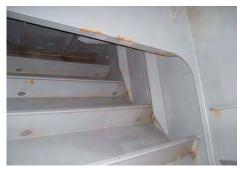
Good condition on welds and sharp edges after
