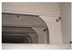
Excellent application properties and final appearance at newbuilding on a ballast tank
