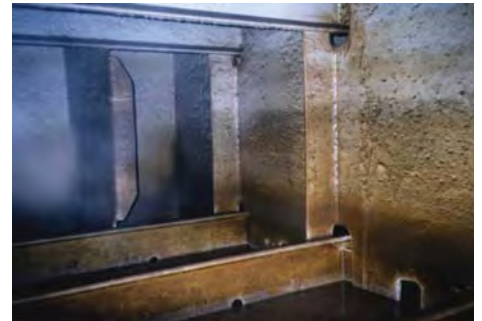
Excellent condition in the water ballast tank after 15 months
