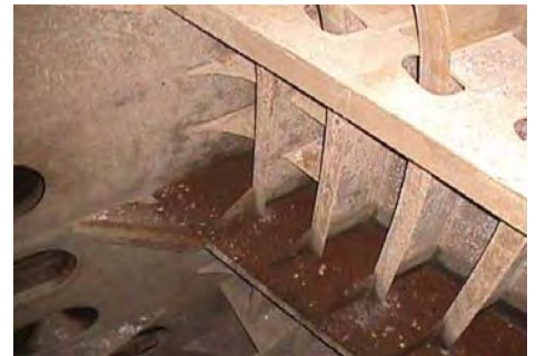
Excellent condition in the water ballast tank after 38 months
