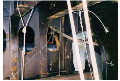
Condition of ballast tanks prior to work commencing
