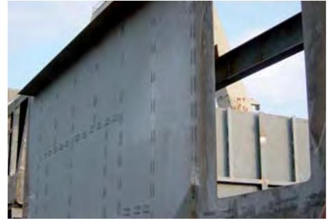
Corrosion protection after heating due to welding processes
