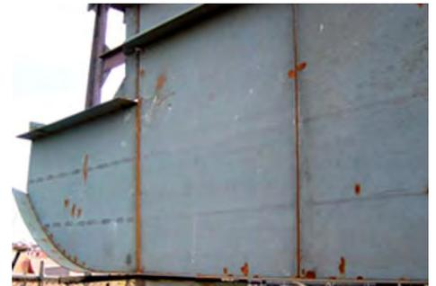
Excellent in service anticorrosion protection even after heating due to welding processes
