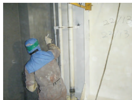
One-coat system reduces number of coats, 1 resulting in improvement of work efficiency at yard.
