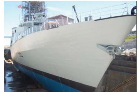
HMCS Charlottetown under major refurbishment, completed with full coat of Interlac®1
