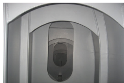
Completed application to the ballast tank areas
