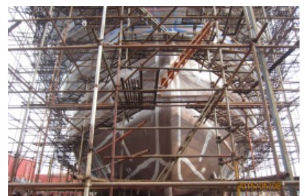
Completed application to the hull part
