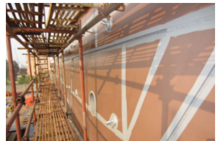
First coat and stripe coat of hull
