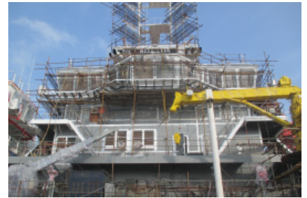
Completed primer application to superstructure
