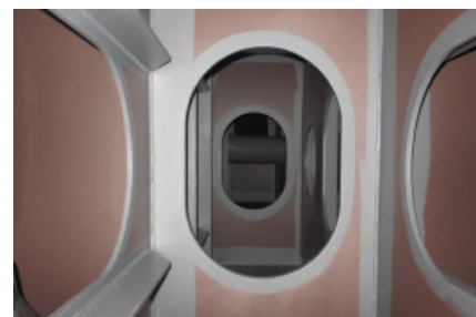
First coat and stripe coat of ballast tank at block stage
