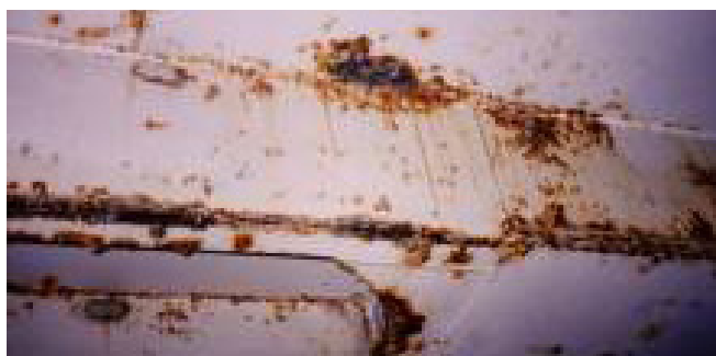
Normal epoxy after 10 years in-service. VLCC
