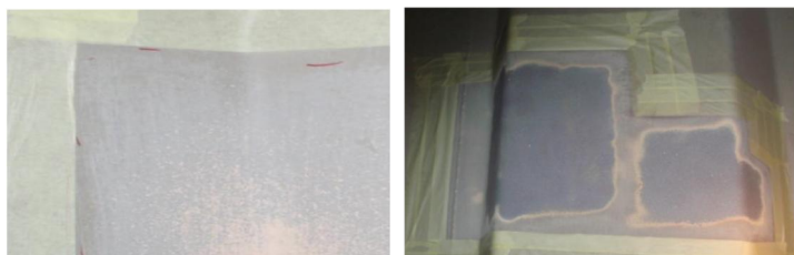
Examples of (1) squared off areas, (2) sanded coating and feathering back of intact coating
