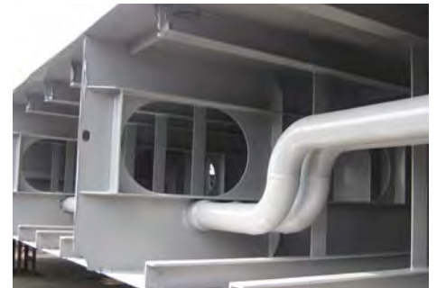
Completed application in the ballast tank of a block section
