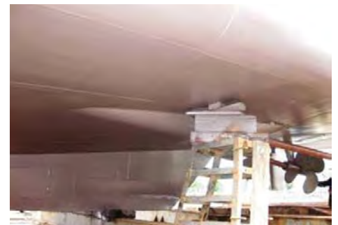
Application to the underwater hull of a patrol vessel
