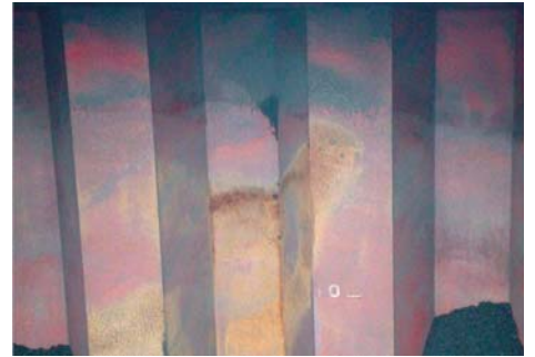
Severe corrosion can quickly follow
