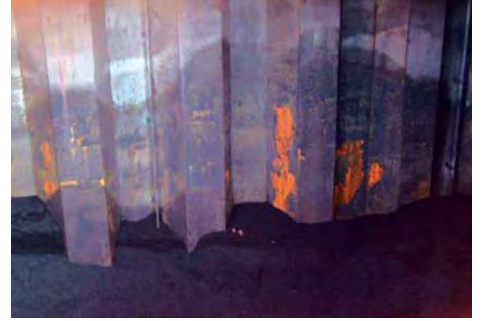
Typical damage from belt conveyor loading
